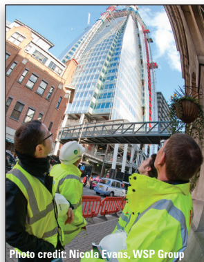
The Shard construction rises above London.
